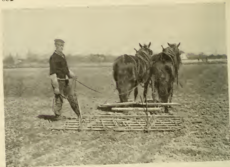
FIG. 145.—Spike-tooth harrow
